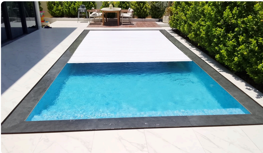
A family pool, cover half open. The roller sits in the water at the far end; nothing was built to take it.
