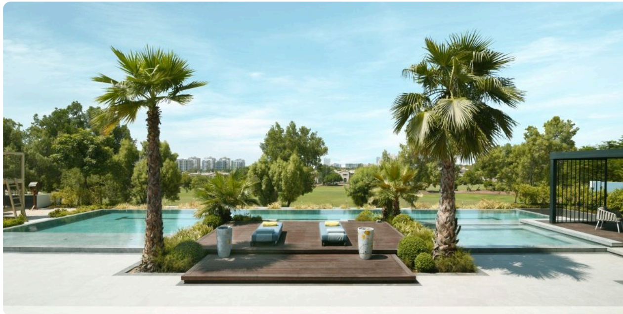
Two pools on one deck, with the plant and treatment behind them sized for both.
